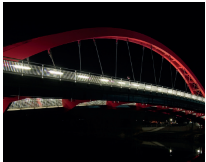
StreamLight 70 - handrail lighting, bridge
